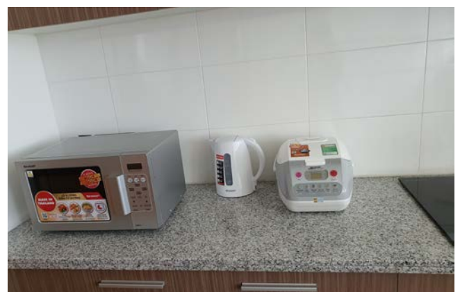
Kitchen appliances installed.
