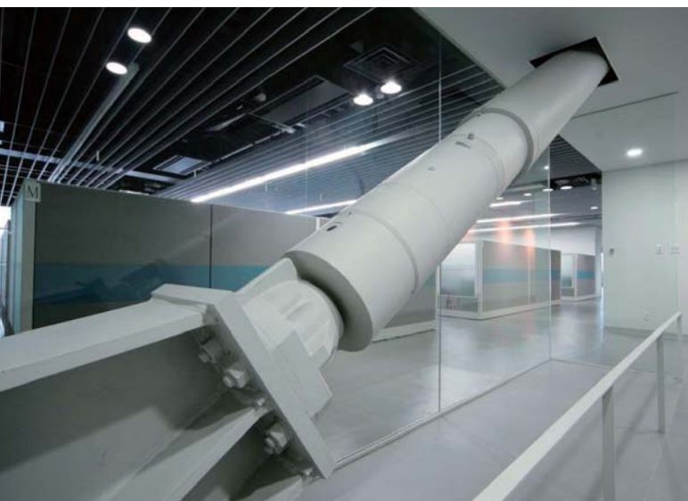
There are approximately 570 seismic dampers inside the plant for absorbing earthquake vibrations
