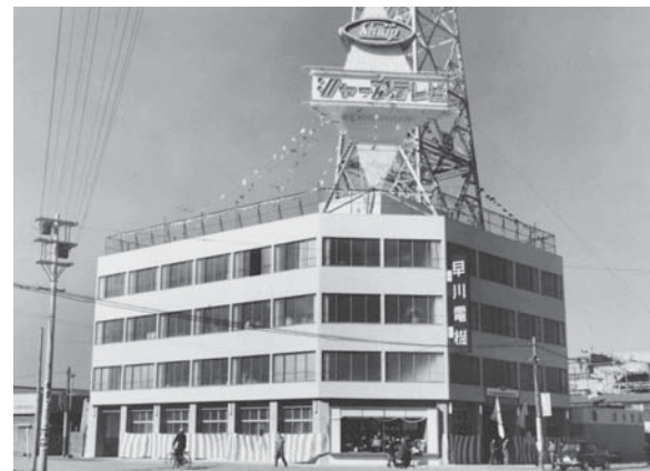
Fukuoka Branch building in Nagahama-cho, Fukuoka City (now Nagahama, Chuo-ku, Fukuoka) (1958)
