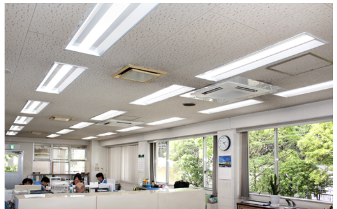
Office lights were changed from florescent lights to embedded LED lights.
