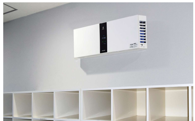
Space saved by installing a wall-mounted unit over lockers.
