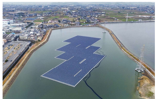
Beautiful installation with consideration to the environment was highly praised.
