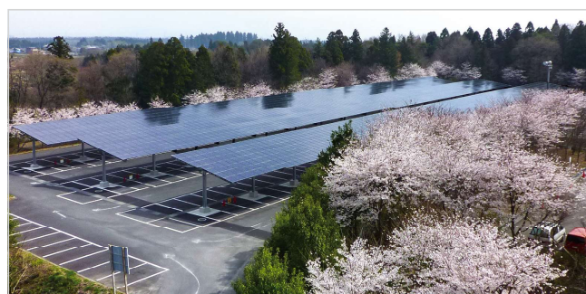
Solar parking with approx. 500kW solar power generation system
