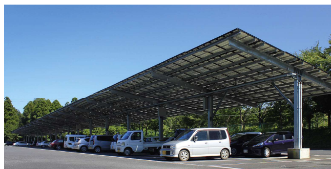
Frame design prevents heat from building up. Maximum power was generated in August 2013.
