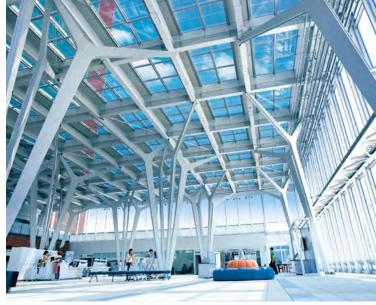
Thin-film, see-through solar modules used in skylights (City Hall, Suzuka City, Mie Prefecture, Japan) (Photo reproduces appearance in clear weather)
