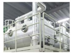
Reducing the volume of washing waste liquid via an evaporator
