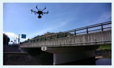
8K-camera drone on an aerial inspection
