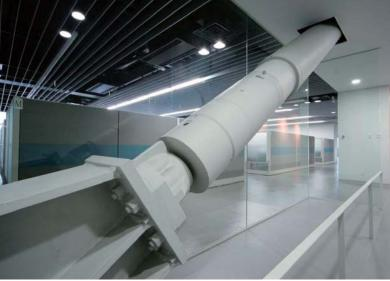
There are approximately 570 seismic dampers inside the plant for absorbing earthquake vibrations
