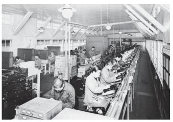
Radio production line using the intermittent belt conveyor system (around 1936)
