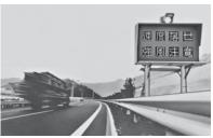
The world's first road weather information system installed on the Tomei Expressway used an illuminated board to automatically display traffic warnings (1969)
