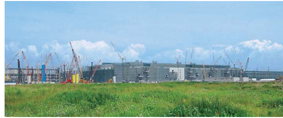
The new LCD panel plant currently under construction (as of July 2008)
