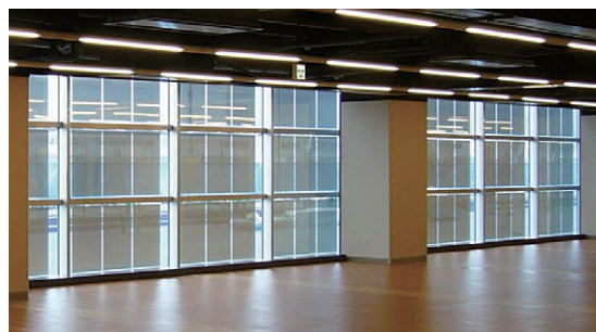
Thin-film see-through solar cells installed at the Kameyama No. 2 Plant (left: external appearance, right: view from inside)
