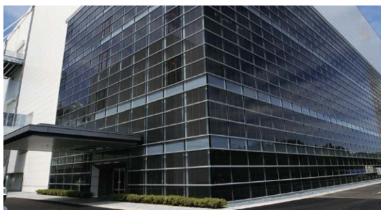
Thin-film see-through solar cells installed at the Kameyama No. 2 Plant (left: external appearance, right: view from inside)
